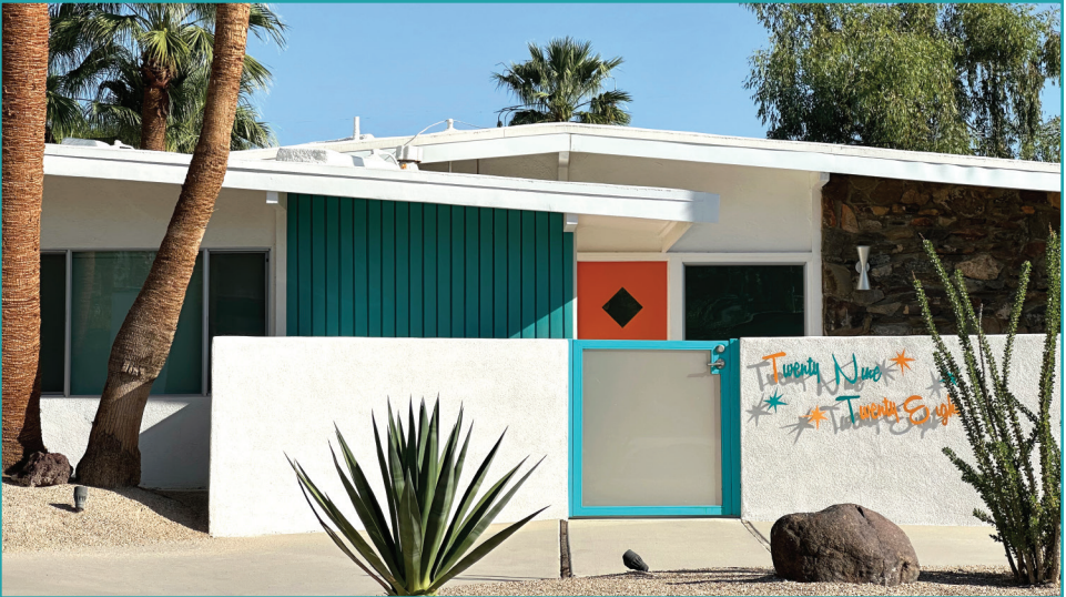
Newly renovated Sunmor mod-pod.
